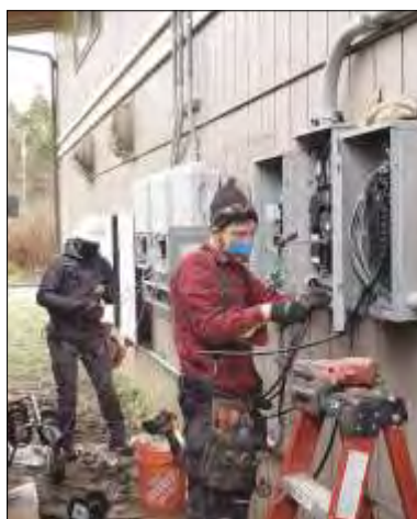
Electricians readying the inverters. Photo by Kelsey Moldenke
